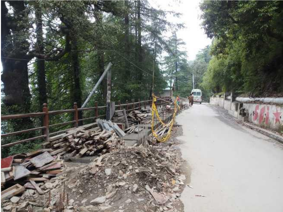
The work on the Sanjauli-IGMC smart path could not start on patches where forest clearance is required.
